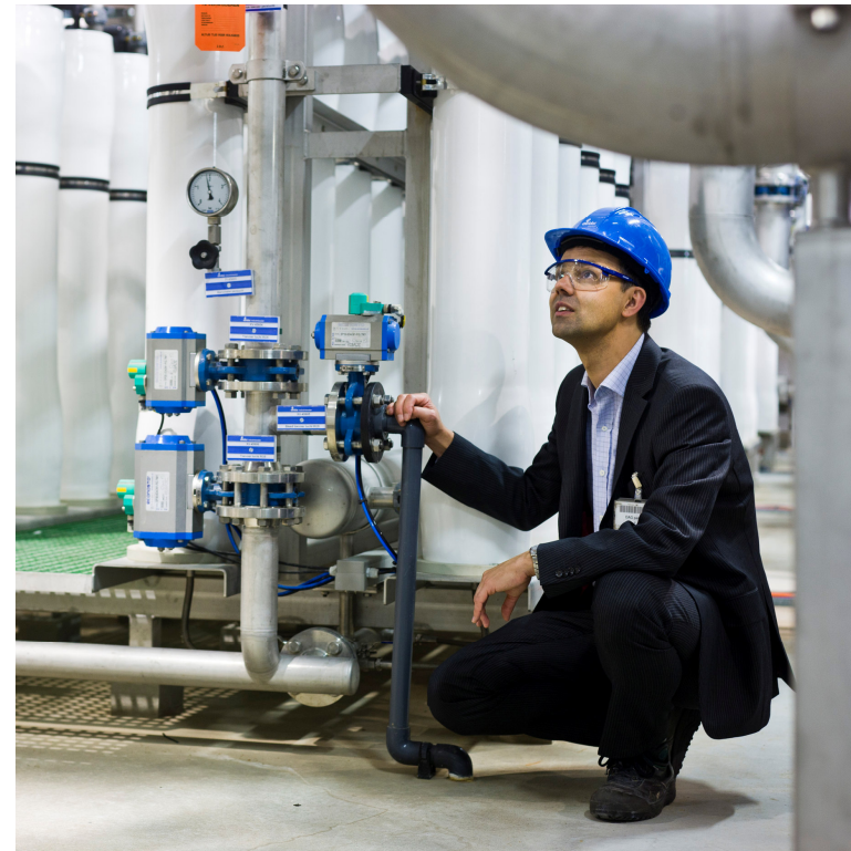
Evides Industriewater, DWP plant (2010) Using AiRO technology developed by KWR Capacity: 1,400 m 3 /h industrial Demi Water Source: Brielse Meer Water
